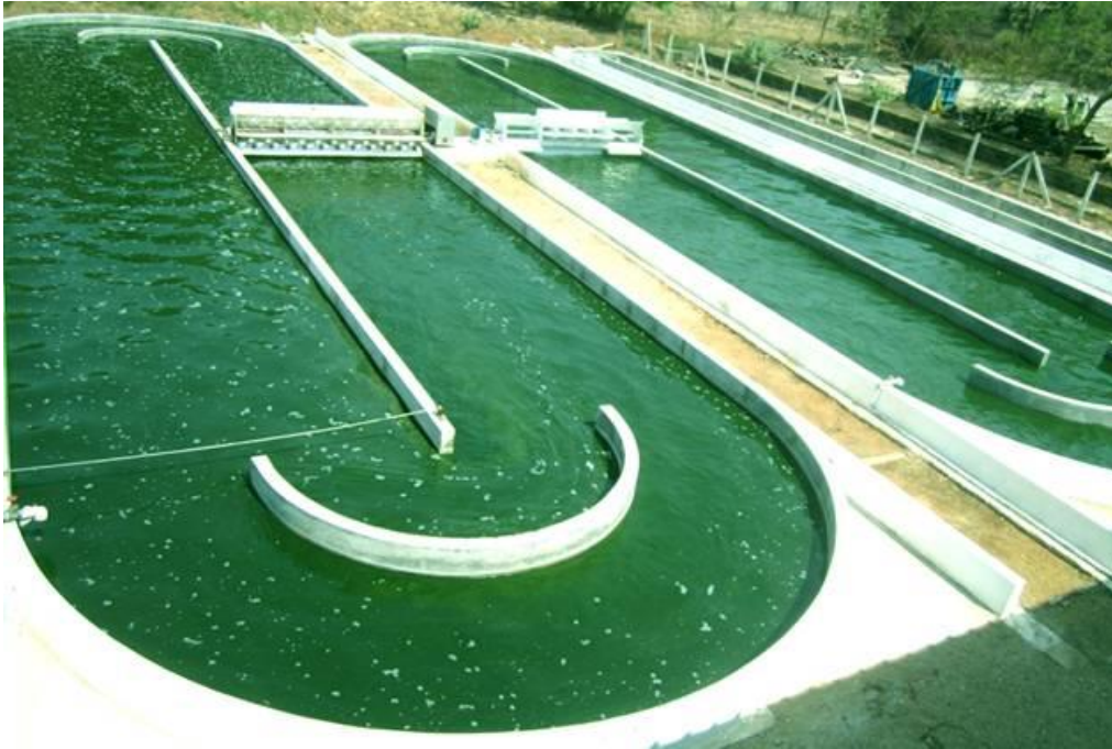
Figure 16 Algae-based wastewater treatment plant at ABAN Bio-tech, Chennai.
